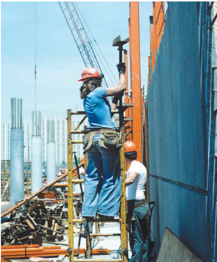
Ladder is placed incorrectly. If possible, worker should be facing operation. This is an unsafe, awkward work posture.
