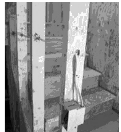
Nonmetallic sheathing helps protect wires from damage.
