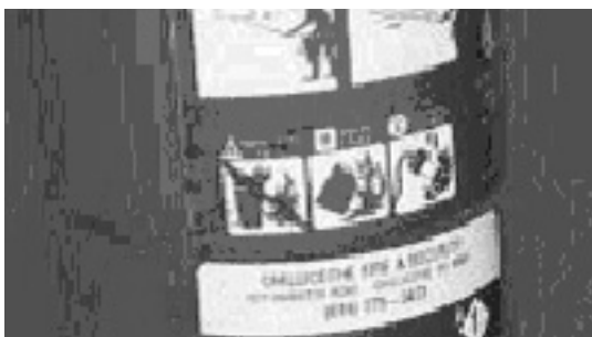
This extinguisher can only be used on Class B and Class C fires.
