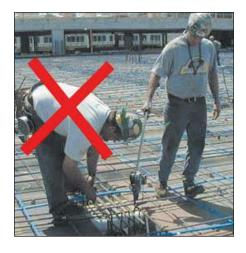
These tying tools also eliminate the risk factors of precise hand and finger work present during the traditional "wire and pliers" method.
