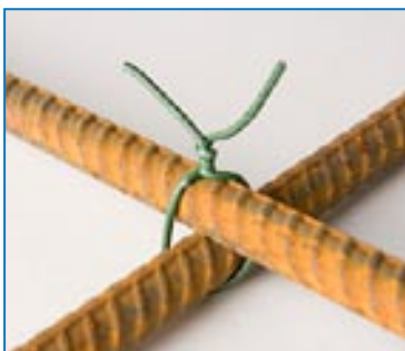
Change technique. Reduce the number of repetitions by not over-twisting the tie. Often a half twist is enough.
